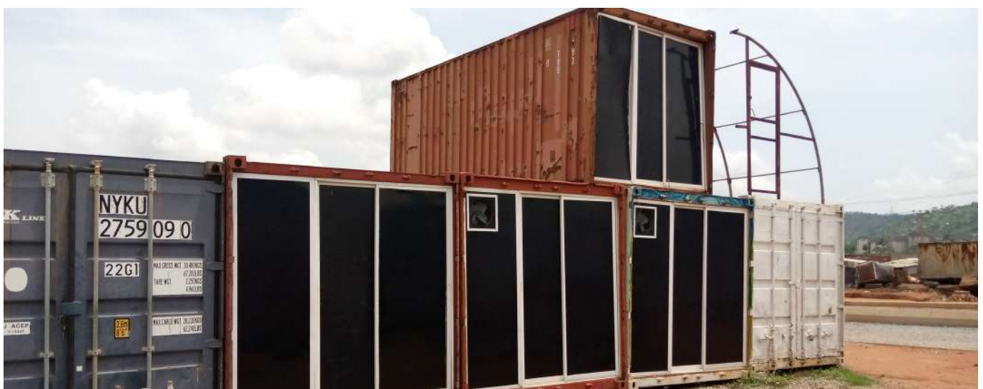
Vertical Farm Using Containers
